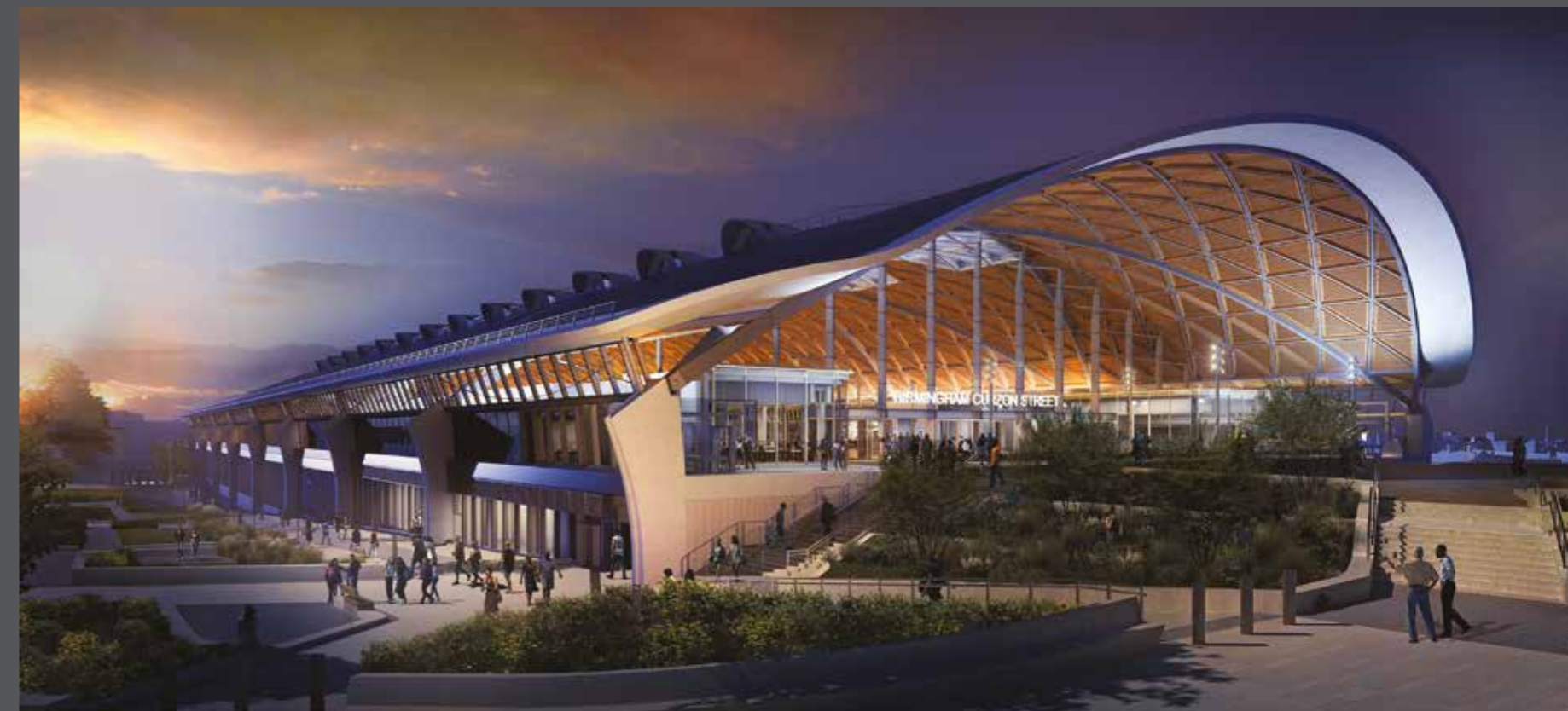
HS2 - BIRMINGHAM CURZON STREET STATION (BIRMINGHAM)
